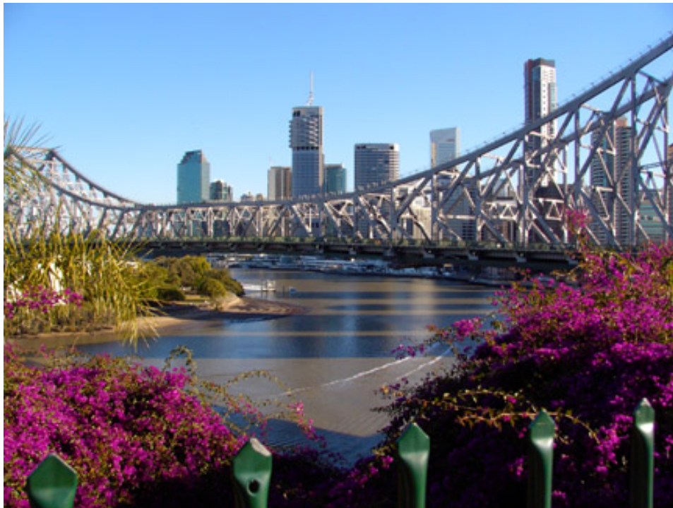
Bridge we cycled across in Brisbane
